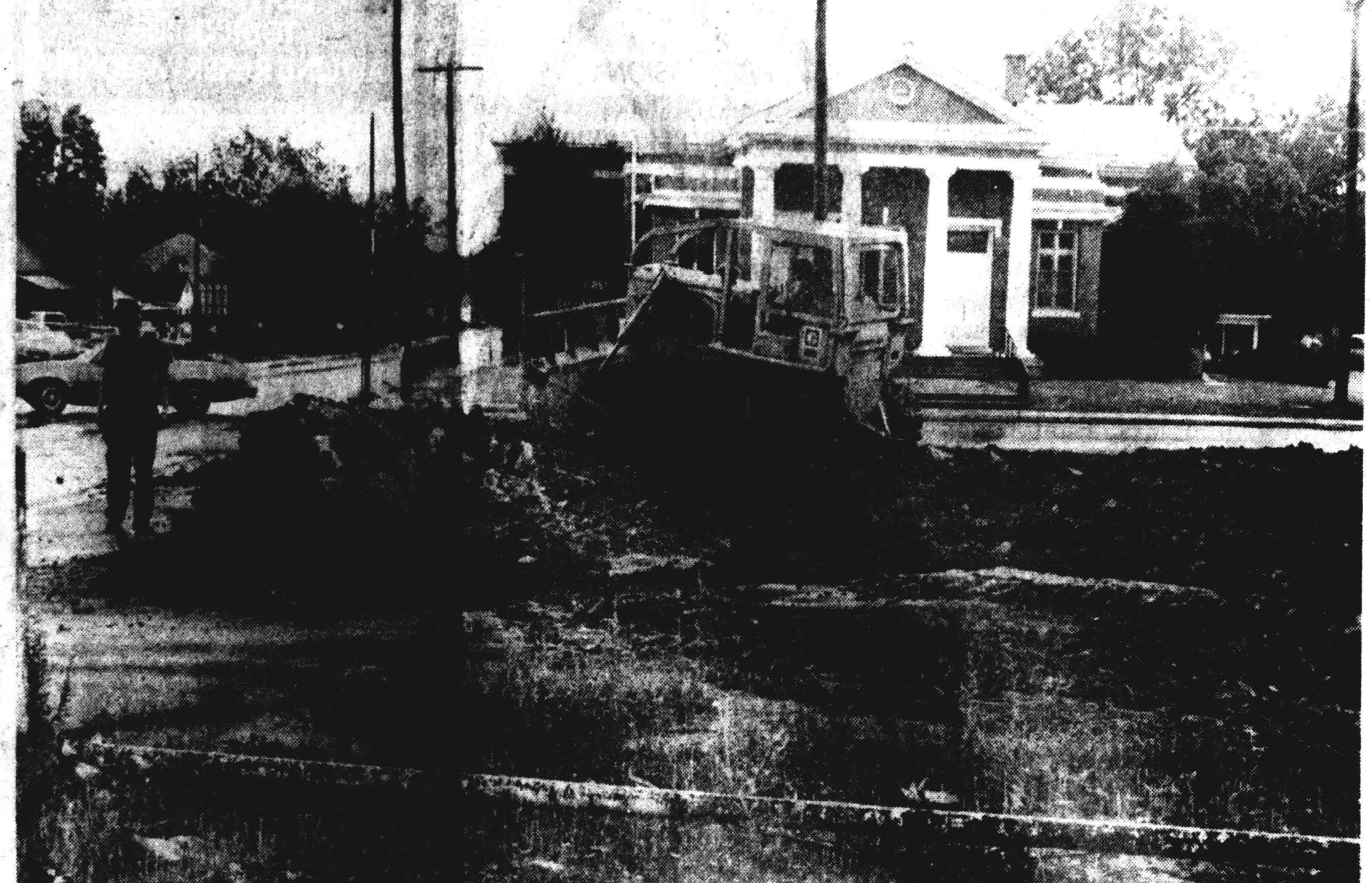
KEY CORNER EXXON service station will be built by John C. Castellaw, of Dyersburg, and Jerry Puckett, of Halls, on lot being leveled at the intersection of Tigrett and Church Sts. in Halls, formerly used by Townsend-Daws/McDearman Ford.
